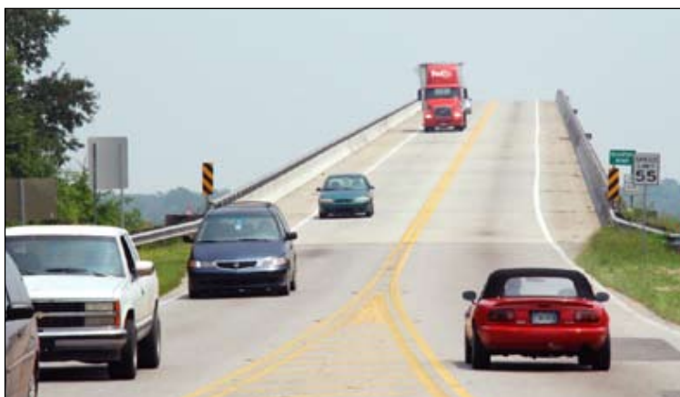
Traffic is back to normal now that repairs to the McTeer Bridge over the Beaufort River have been completed. The bridge was damaged by a barge back in April.
