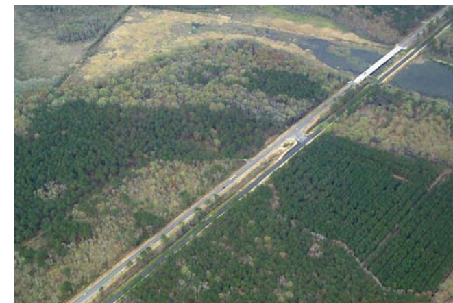
Aerial photo of Segment 1 Phase 1 with the intermediate and surface paving completed between the Combahee River and Jacob White Road.
