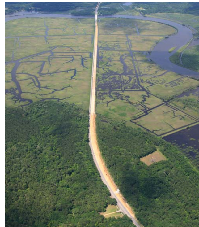
Aerial photo of Segment 2A
