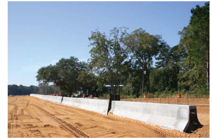
A permanent barrier wall, placed within the Gardens Corner interchange, separates the frontage road and a new US 17 lane, which will take southbound US 17 motorists to a new roundabout with access to US 21.
